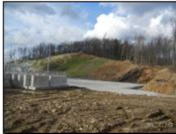
98 MW Wind/32 MW Storage Project, WV-US (in construction)
